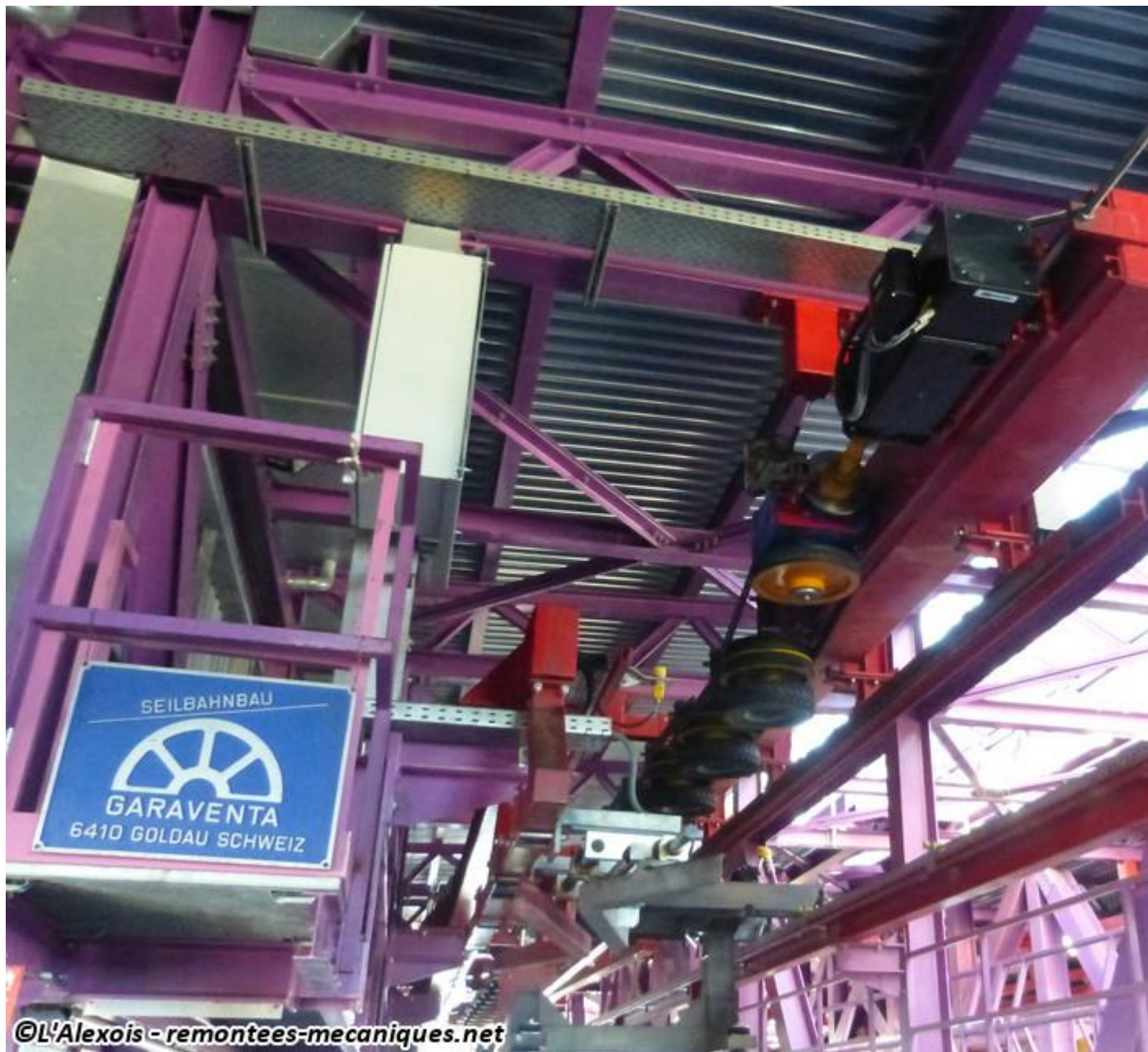
Speed reducer motor in the upper station
