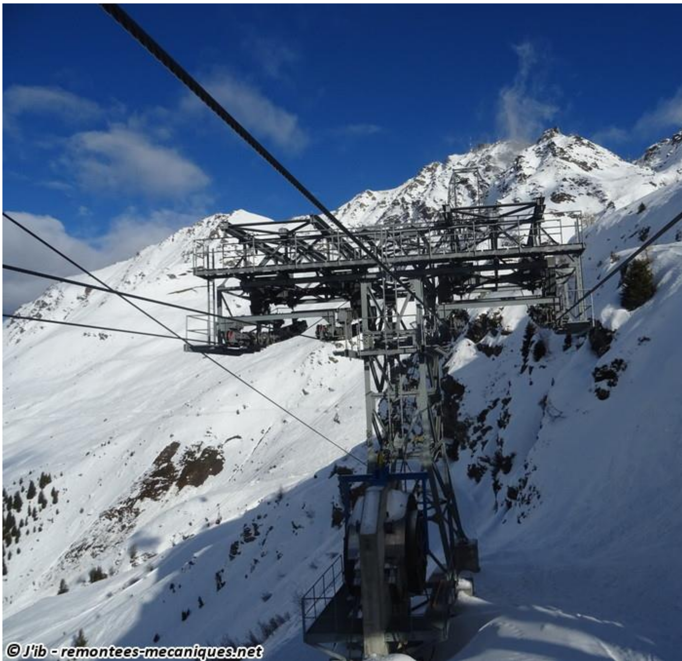
First pylon. Unlike Montana, this compression pylon is not linked to the departure station. This is explained by the fact that the line had to remain low enough at the exit of the station for the TCD4 of Attelas to be able to fly over it.
