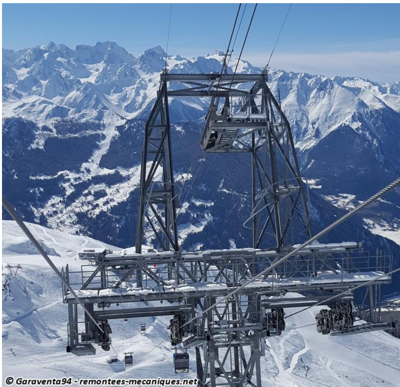
The shoe on the P3 from above
