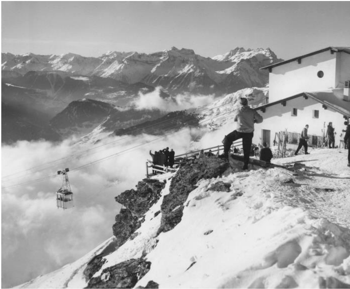
Les Attelas probably in the winter of 1958. We can observe the deviation of the carrying cables going beyond the station to be fixed around an anchor plate cast on the ground. (François Luisier Collection)
